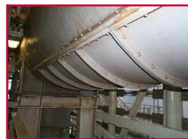
Three years on & the installed PFP system is performing well offshore
